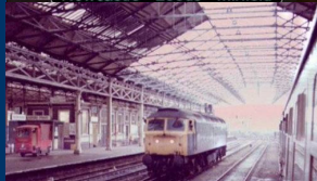
Section: 2 Huddersfield - Liverpool Lime St
